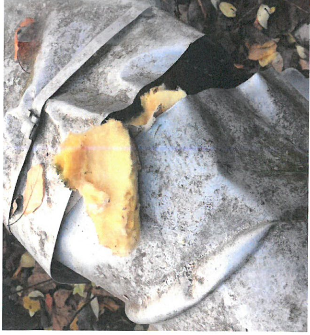
Photo 3 – A view of the fiberglass insulation on facility piping.
