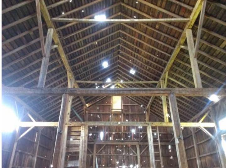
***“Due to the extreme wear and damage to the roof and the North wall of the barn, we removed all interior items, metal fixtures and exterior siding first. Then, after further assessment, we strategically pulled the structure down to ground level.” – Holly Reed***
