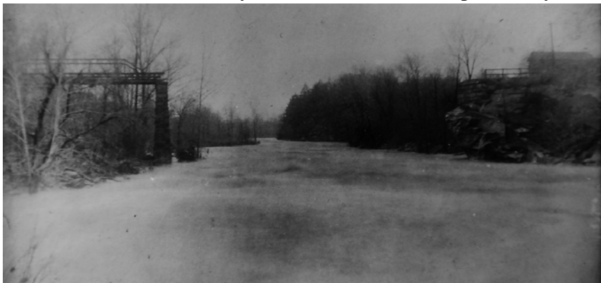
The March 25, 1913, flood knocked out most of the bridge, but the stone pillar near the west bank remained standing. Part of that pillar still stands today below the current bridge.
