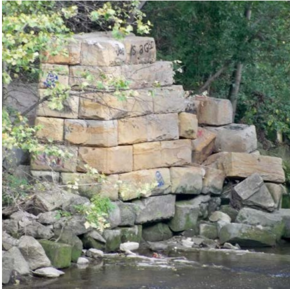
This portion of the stone pillar Gib Doolittle built near the west bank of the river in 1864 remains underneath the current bridge.
