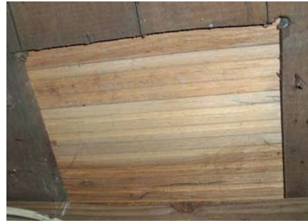
Oak flooring for the first story shows through the older poplar boards in the basement ceiling.
