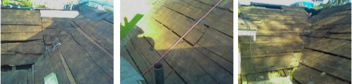
These photos show the wide plank boards that were revealed when the roof was removed in the fall of 2008. Photos courtesy of Kevin Roberts.
